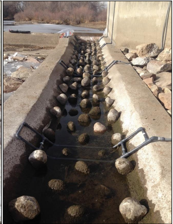
Figure 1.2- Top photo shows the Fossil Creek Inlet Diversion low head concrete dam including the fish passage on the far right and the radial and ditch gates on the far left. Bottom left shows the inner configuration of the fish passage, with trapezoidal cross section and cobble roughness elements. Bottom right shows the antenna placement (grey pipes) within the passage.
