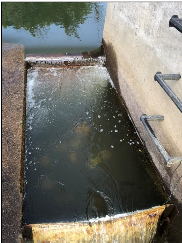
Figure 2.7- Top left (A) photo shows the design and day to day operating conditions of the Rough and Ready/Palmerton site's pool-weir-and-orifice style fishway. Bottom right (B) photo includes the temporary replacement weir plates used during the trial and the lower enclosure box set into the channel exit. At bottom left (C) is shown the checkboards used both to control flow and to act as a top box during the trial.
