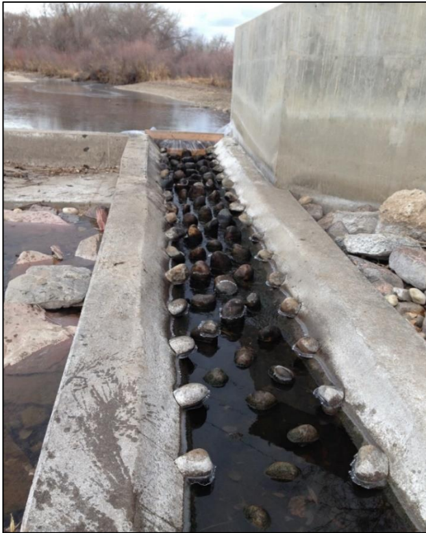
Figure 1.2- Top photo shows the Fossil Creek Inlet Diversion low head concrete dam including the fish passage on the far right and the radial and ditch gates on the far left. Bottom left shows the inner configuration of the fish passage, with trapezoidal cross section and cobble roughness elements. Bottom right shows the antenna placement (grey pipes) within the passage.
