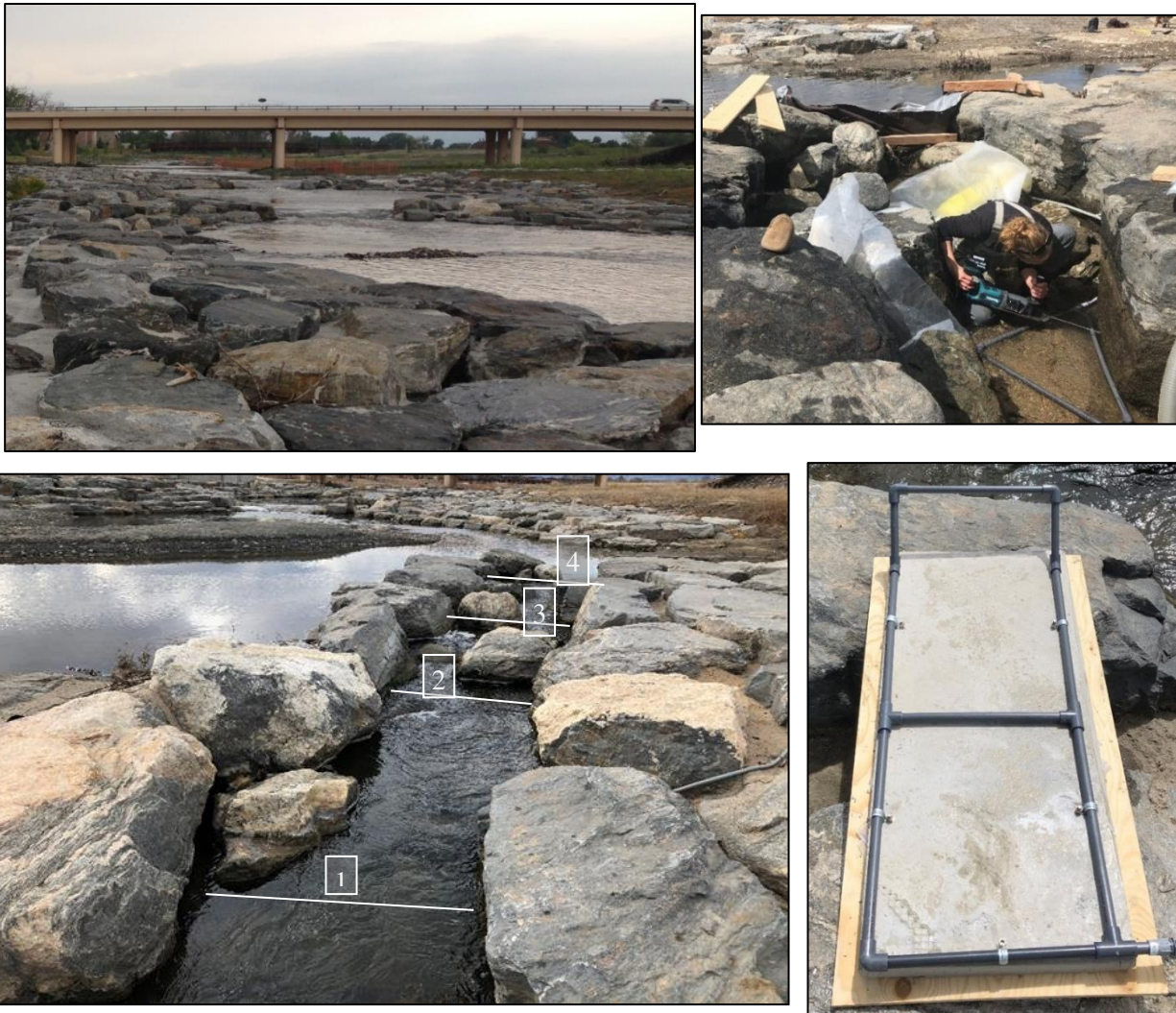
Figure 1.3- Top left shows the downstream-most portion of the Dickens Farm Natural Area, including grouted boulder pool drops, grouted boulder wingwall bypass fish passages on the left side terraces and bank stabilization. A closeup of the studied passage structure is shown at the bottom left, with the locations of the four antennas denoted by red lines. Photos to the top and bottom right illustrate the various approaches taken to secure the antennas in the passage for the duration of the study.
