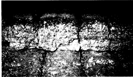
Figure 3.33 Interlocking Joints between Blocks
