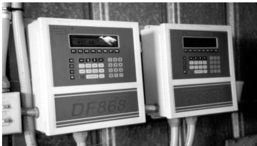
Figure 4. Digital display screens for new Panametrics flow meters inside the Portuguese Bend pumping plant.
