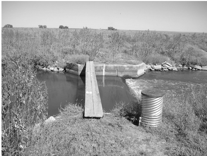
Figure 2. Riverside Irrigation District has several rated sections with wet wells available for WSL sensors.
